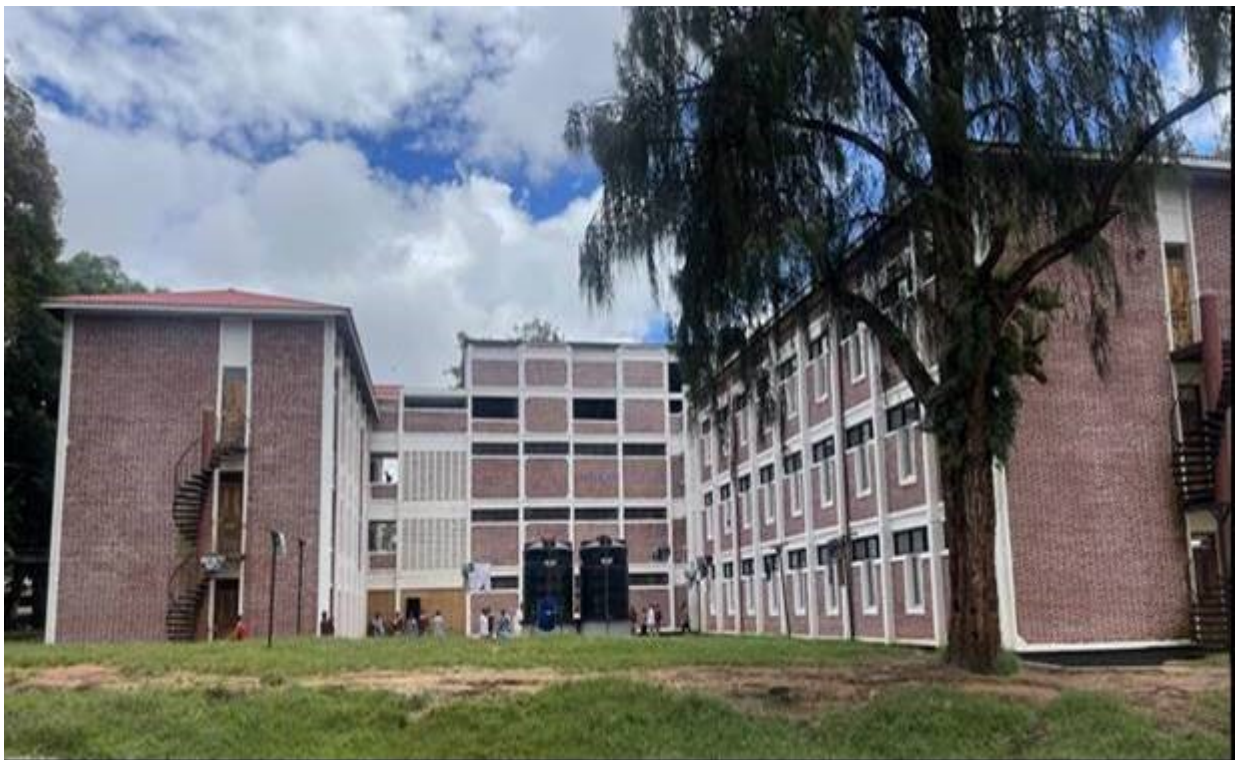
Figure 2.3: Njombe Secondary School
