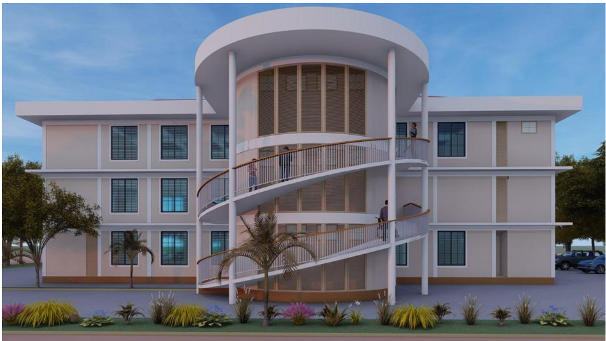
Figure 2.3: Rear view of the building
