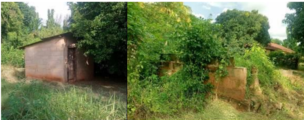
Plate 2.3: Existing structures in site
