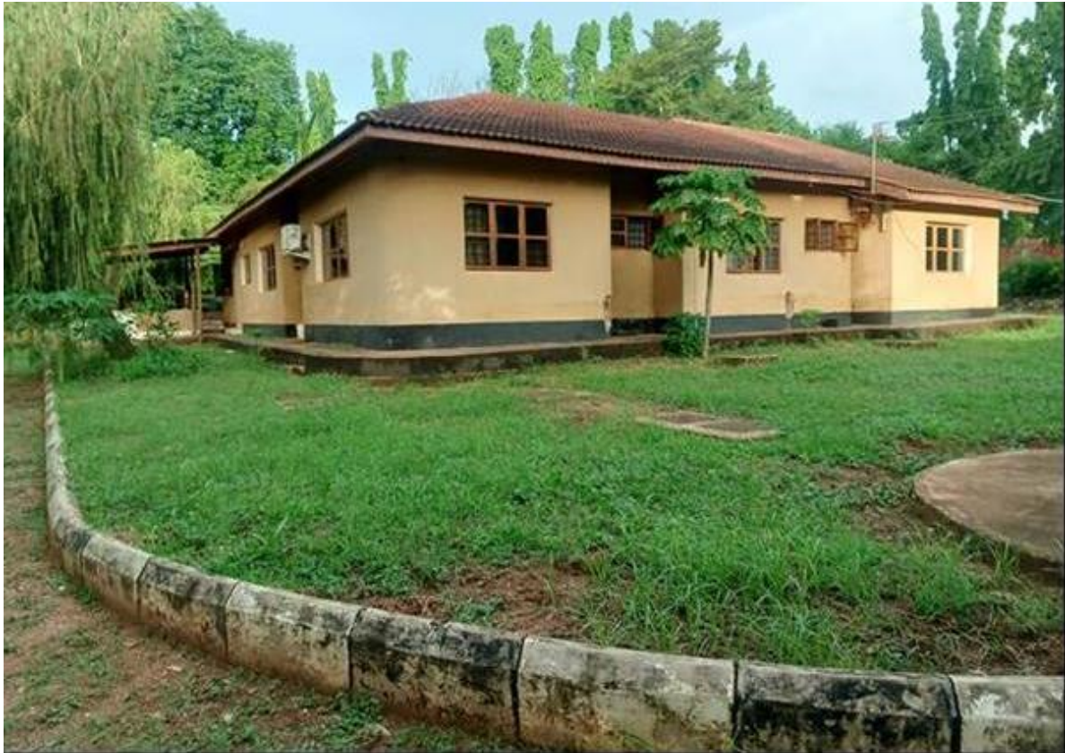
Plate 2.2: The Main building (OUT Regional Centre Office)
