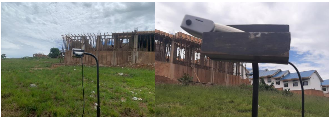
Figure 4-4: Ambient Air Quality Monitoring equipment used at the project site (Tansheq Site Visit, November 2022)
