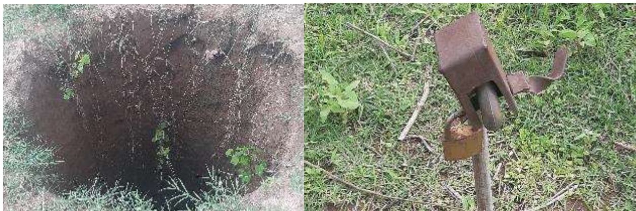
Figure 4-8: Water infrastructure on site which is distributed water taps (Source: Tansheq, 2023)
