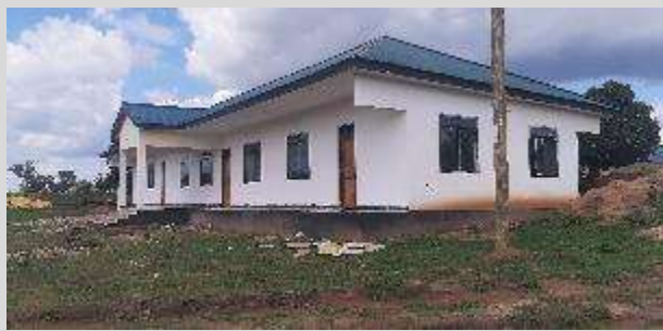
Figure 4-2: Secondary school constructed under SEQUIP (Source: Tansheq, 2023)
