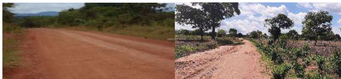
Figure 4-11: Some of passable roads within Nsimbo DC
